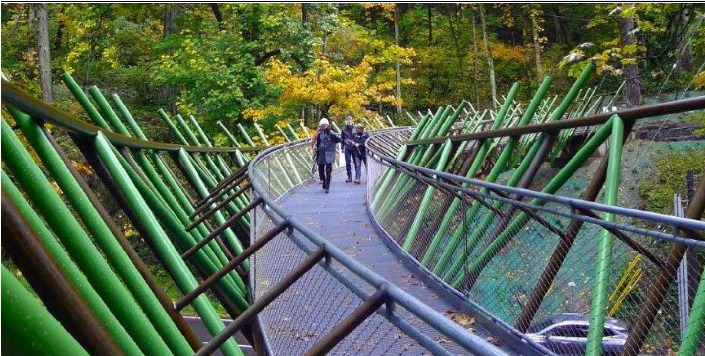
Photo courtesy of Ed Carpenter, Wildwood Trail Bridge at Barbara Walker Crossing The bridge, designed by local Oregon artist, Ed Carpenter, is 178' long measured at the center of its curving deck. Its basic structure is a tri-chord truss of rusting and painted steel. Carpenter's design evokes imagery of the sword ferns and vine maples lining the entire length of the Wildwood Trail. This project is a collaborative effort of the Portland Parks Foundation in partnership with Portland Parks & Recreation (PP&R), the Portland Bureau of Transportation (PBOT), and Metro. Albina Co., Inc. bent 3½" SCH80 A847 and 5" SCH40 A847 all rolled to various radii, as well as 1" SCH40 A53B, 1½" SCH40 A53B, 1½" SCH80 A53B all rolled to various radii.
